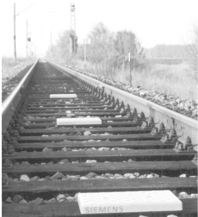
Figure 13.19 Euro balise in practical operation (reproduced by permission of Siemens Verkehrstechnik, Braunschweig)
